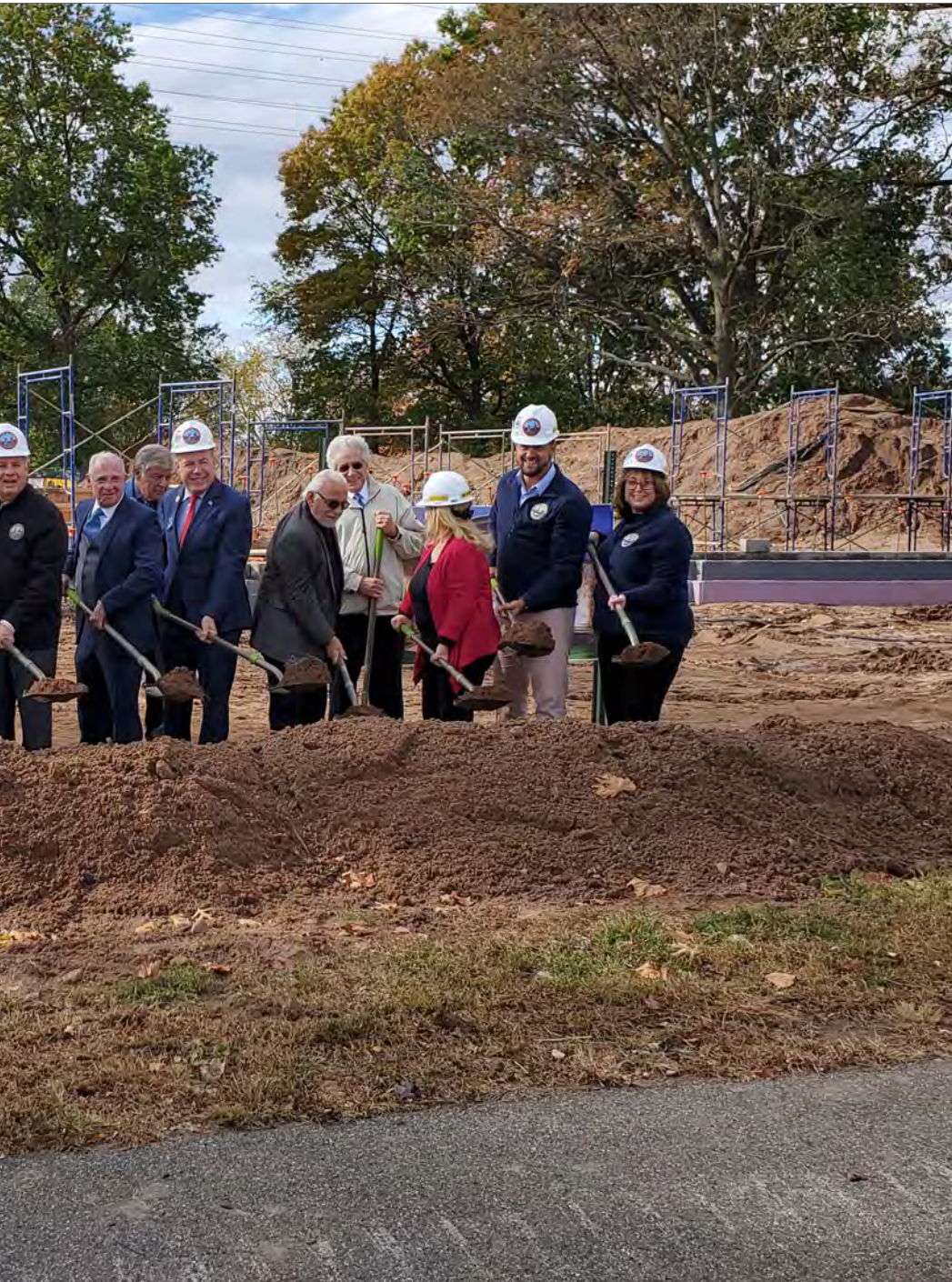
Groundbreaking Ceremony for New Amphitheater and Comfort Station in Riverside County Park in North Arlington Source: Bergen County
