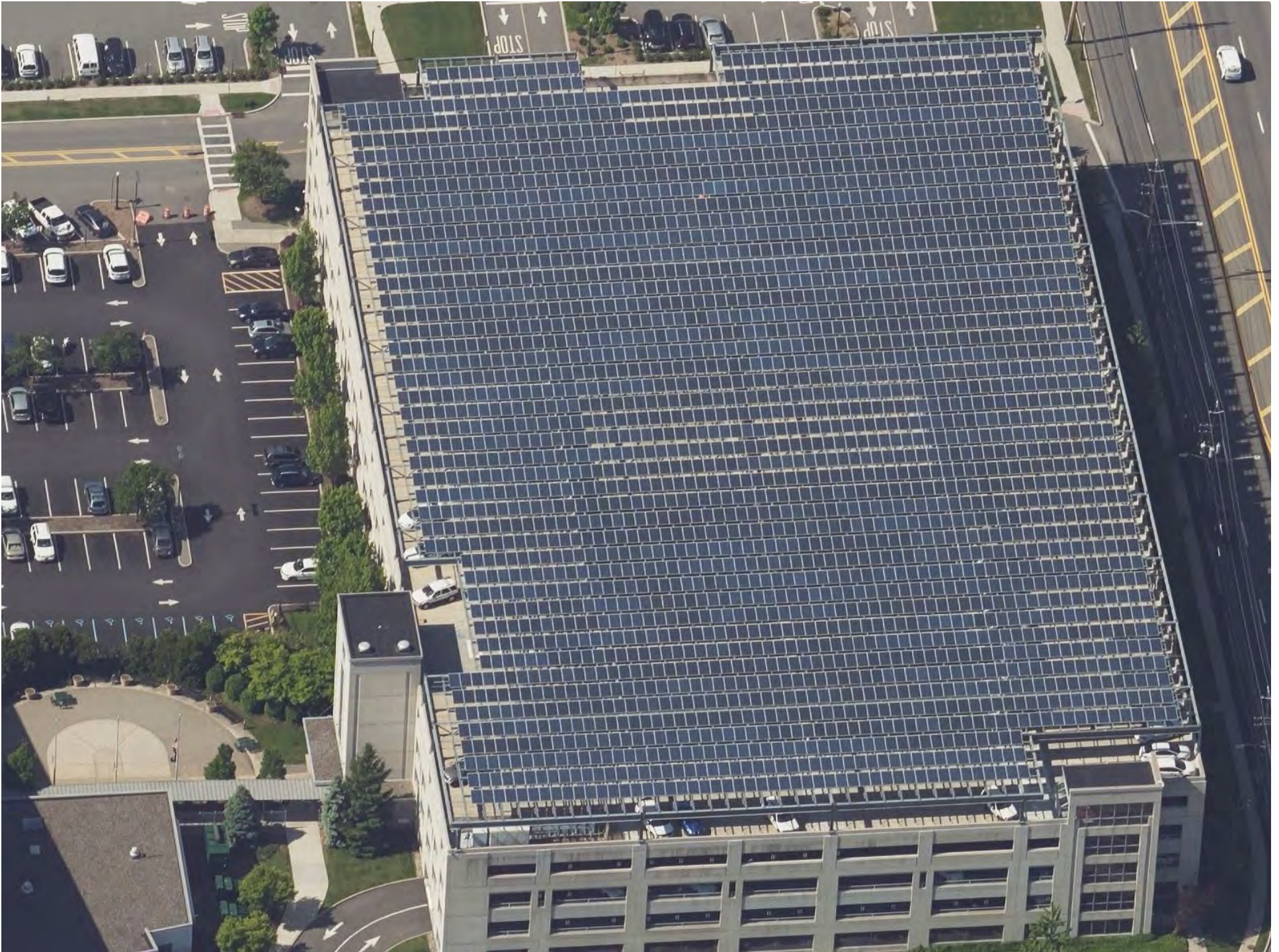
Solar Above County Parking Deck: Source: Bing Maps
