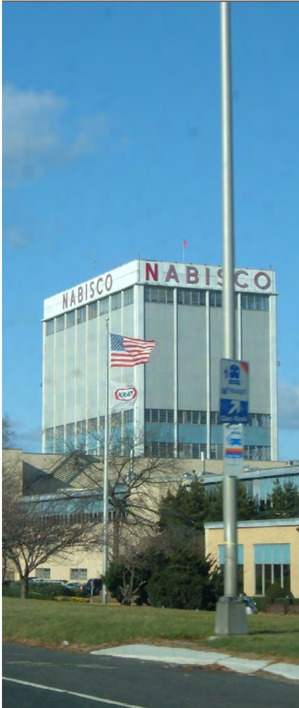
Former Nabisco Plant in Fair Lawn. Source: Colliers Engineering & Design
