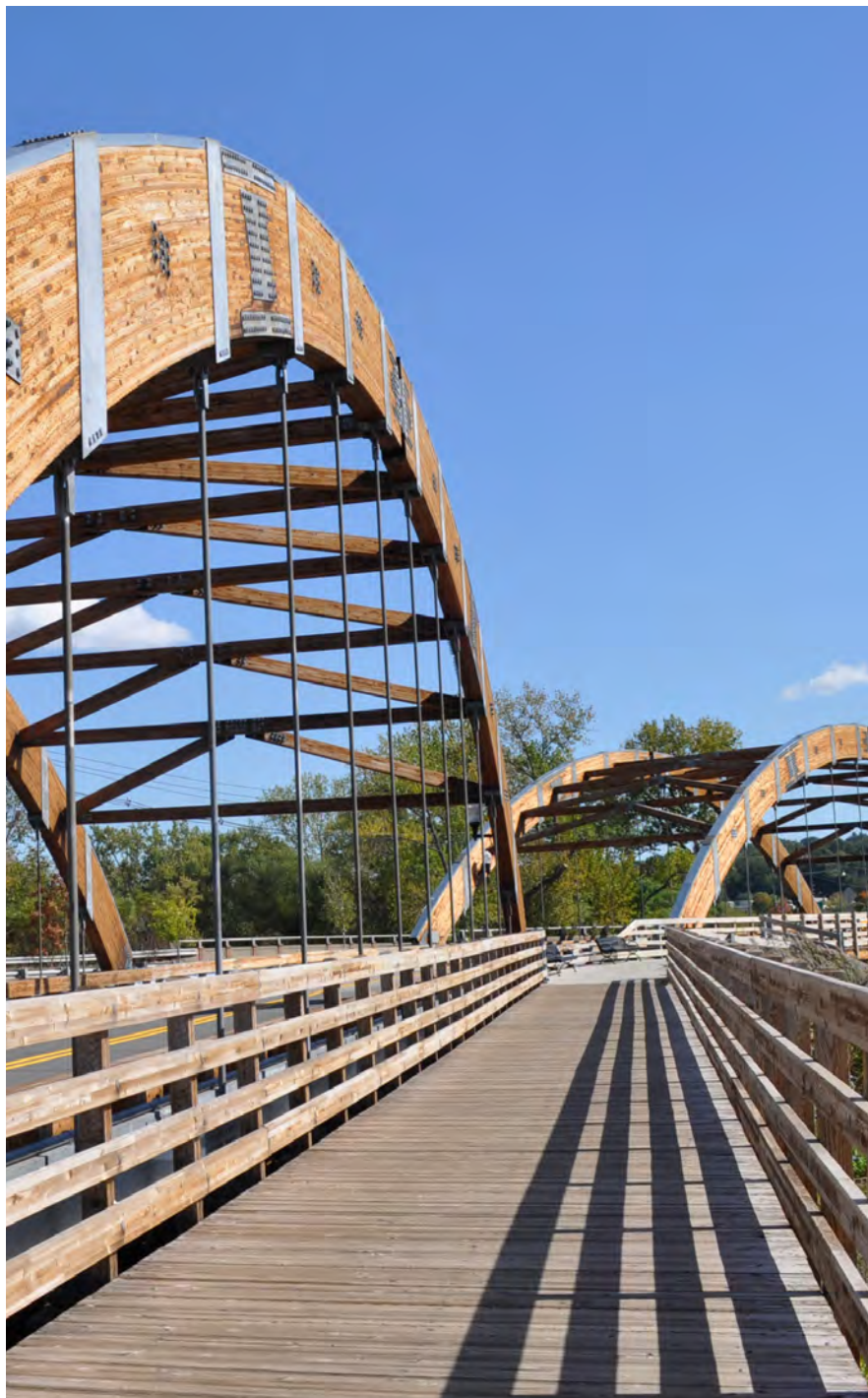
Overpeck Park Bridge. Source: Bergen County Division of Economic Development
