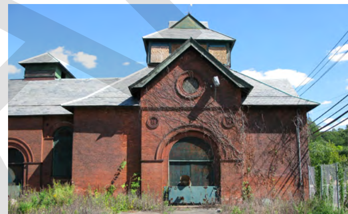
Figure 5. Hackensack Water Works and Van Buskirk Island (Courtesy of CUES)
