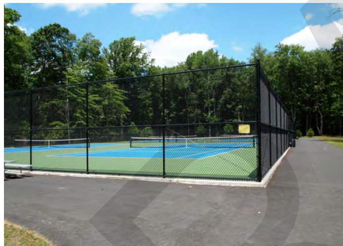
Figure 3. Tennis courts at Wood Dale County Park (Courtesy of CUES).
