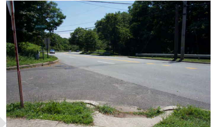
Figure 5. Improving linkages between neighborhoods and nearby parks could facilitate bike and pedestrian access to some parks. In this case, the sidewalk ends at Dunker Hook Road without crosswalks to facilitate easy access to Saddle River County Parks (Courtesy of CUES).
