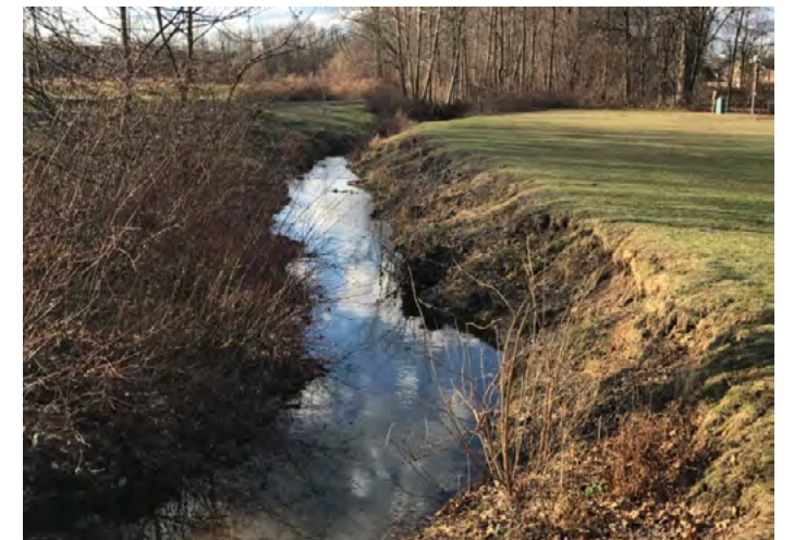
Figure 5. Rockleigh Golf Course streambank erosion in march, 2017 (Courtesy of Biohabitats).
