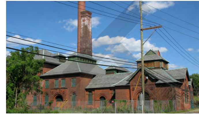
Figure 7. The Hackensack River Waterworks has national historic significance and great potential for vibrant re-use (Courtesy of CUES).
