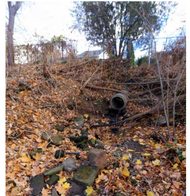
Figure 8. Outfall on steep grade contributes to erosion at Van Saun County Park (Courtesy of Biohabitats).
