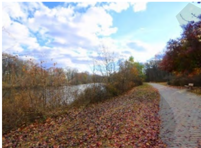
Figure 10. Limited vegetative buffer do not provide enough root protection, increasing the risk of stream bank erosion (Courtesy of Biohabitats).
