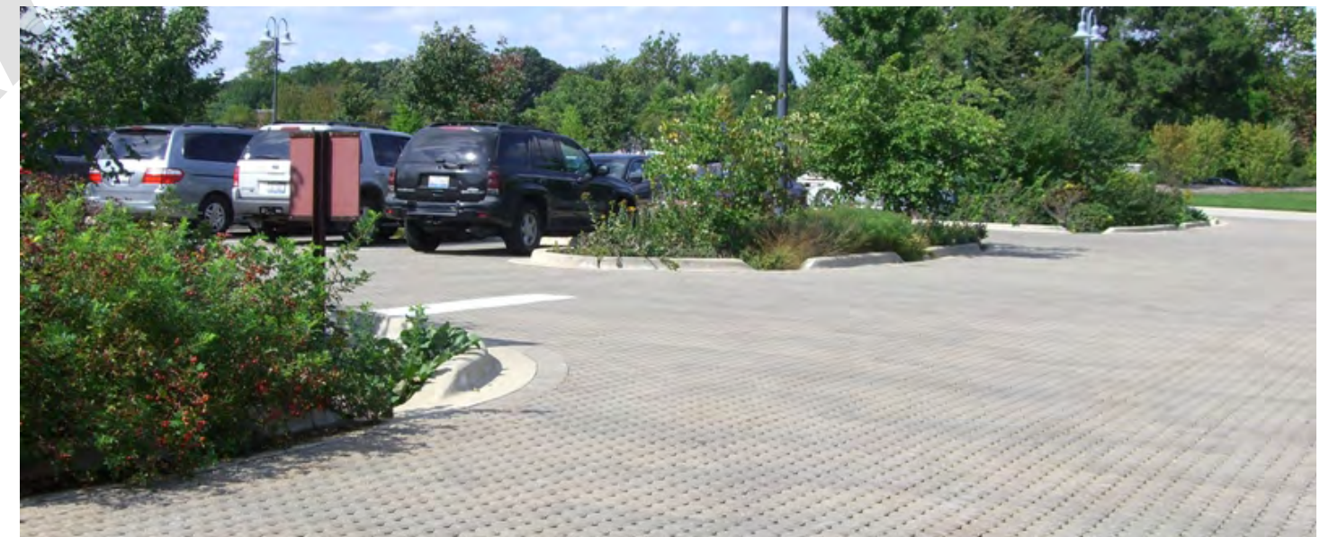
Figure 22. Implementing stormwater best management practices, like the parking lot rain gardens above, can protect and enhance the ecological health of natural resources in the parks, as well as improve user experience (Courtesy of Biohabitats).
