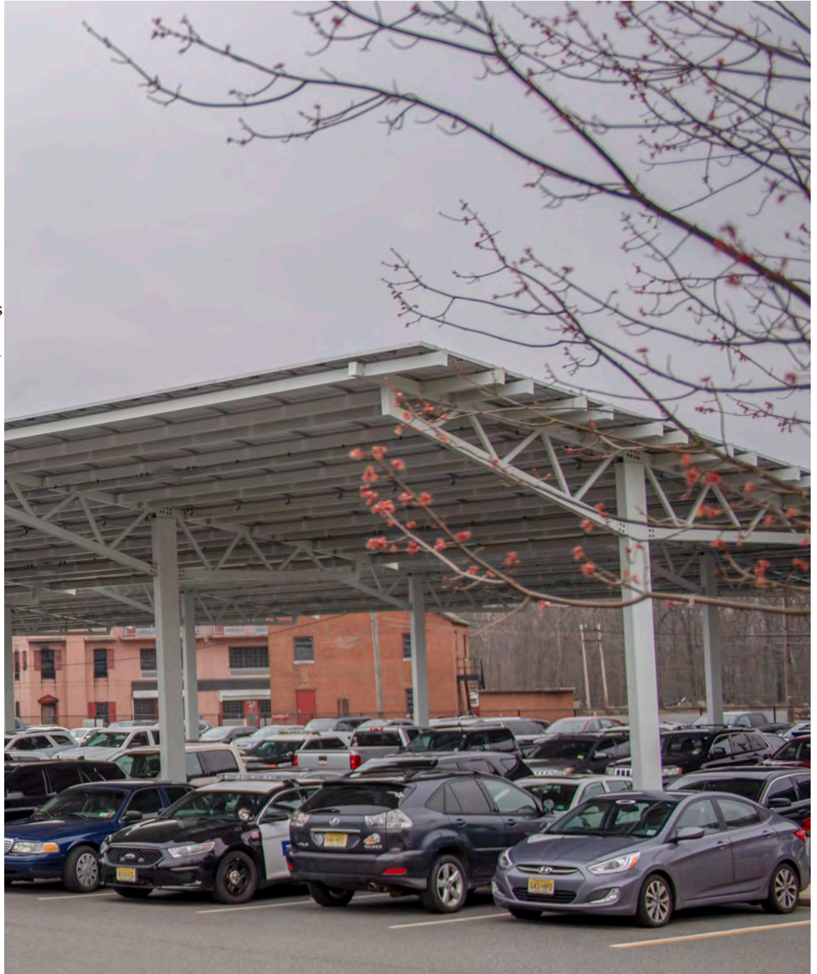
Solar Parking Canopy. Source: Donna Brennan, Bergen County
