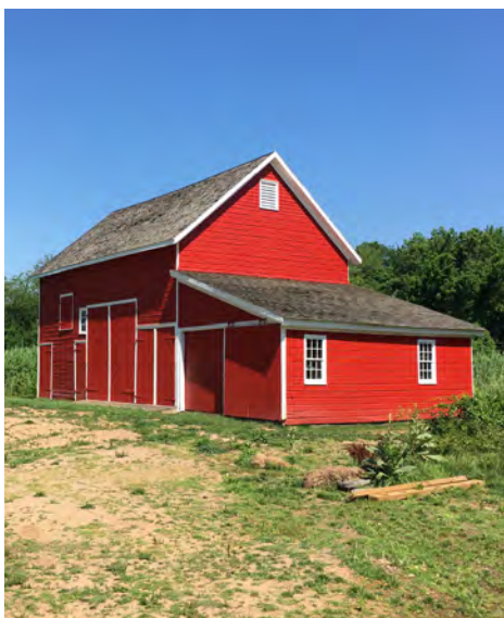
Historic New Bridge Landing Park (Image 3.6.1)
