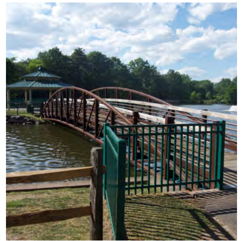
A bridge to the pavilion (Image 3.3.8.3)
