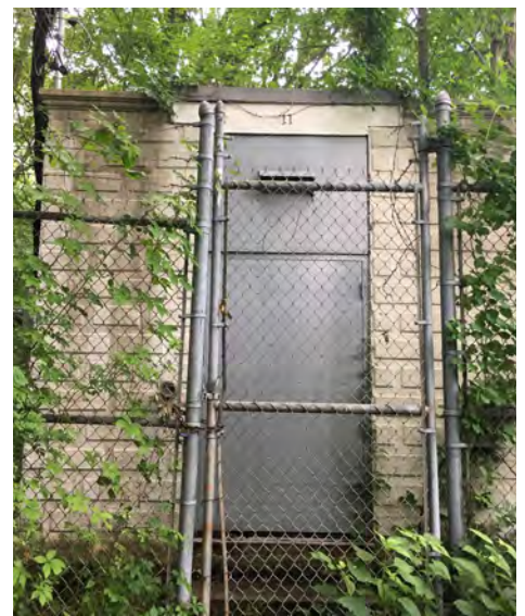
Maintenance structure (Image 3.3.9.4)
