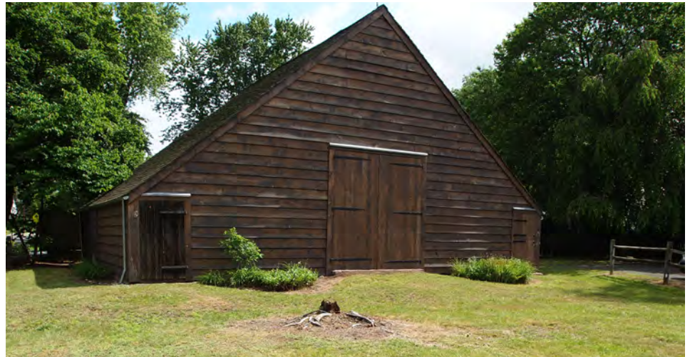
Wortendyke Barn is an excellent example of the vernacular architecture of 18th century Bergen County (Image 3.6.5.1)
