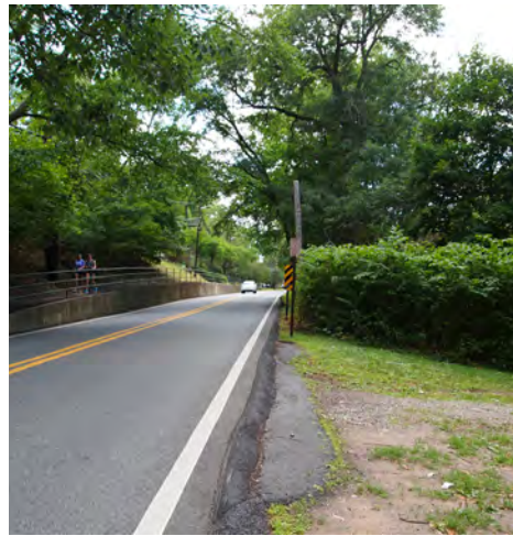
Large curb separates street from entrance (Image 3.4.5.2)
