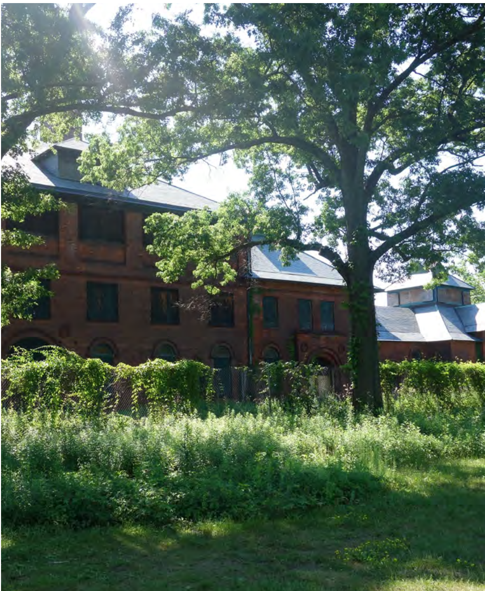
Hackensack Water Works facility (Image 3.6.1.3)
