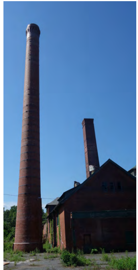
Water filtration towers (Image 3.6.1.1)
