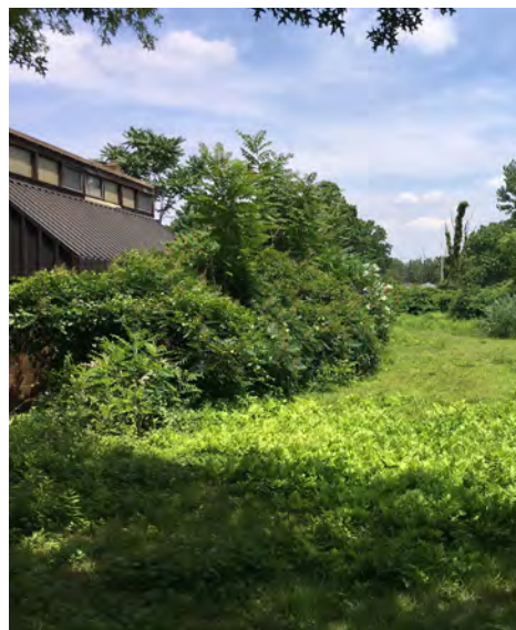
Overgrown building and invasive species area (Image 3.1.2.5.4)
