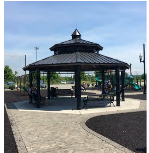
Typical pavilion in playground (Image 3.1.2.2.9)
