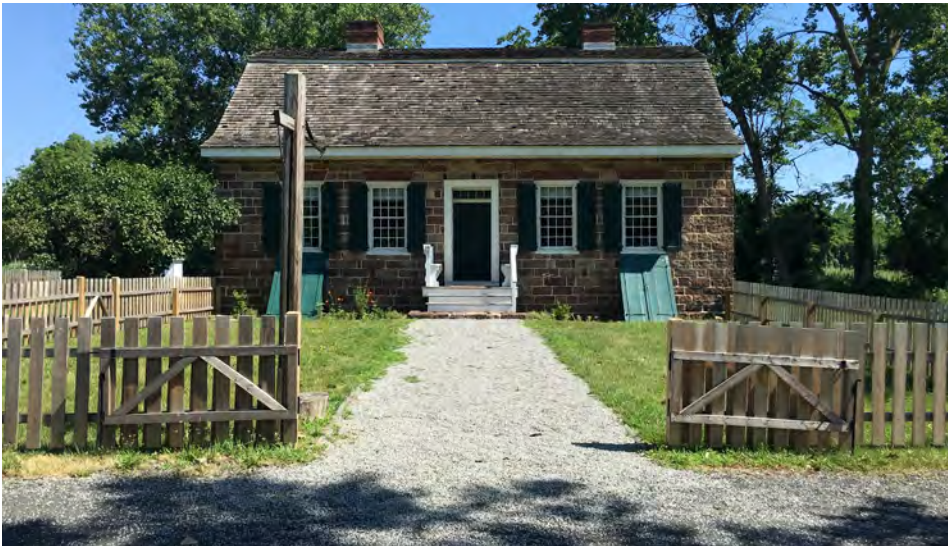
The Campbell-Christie House is the only building owned by the county. (Image 3.6.3.2)
