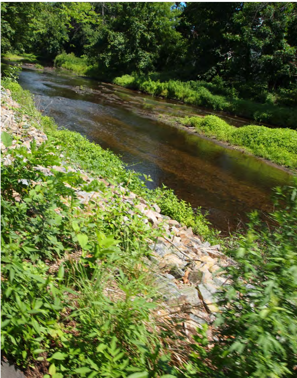
Bank Stabilization (Image 3.1.1.5.2)
