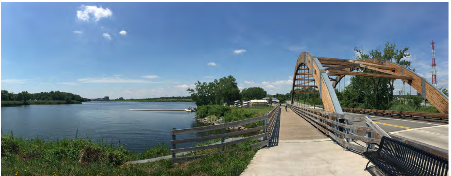
Bridge to northern entrance of Overpeck Area 3 (Image 3.1.2.2.2)
