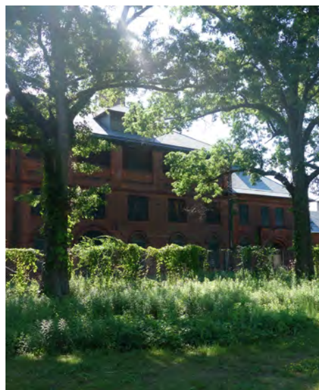
Hackensack Water Works (Images 3.6.4)
