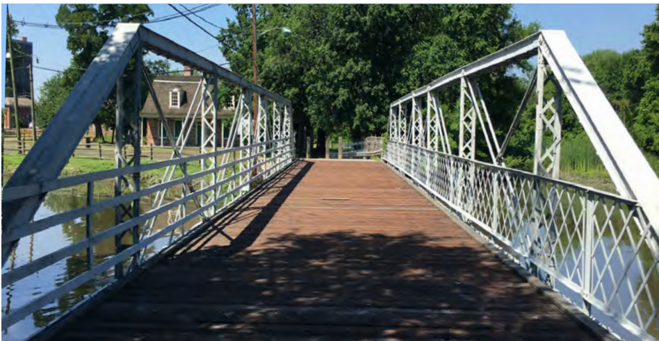
The county-owned bridge looking into the park (Image 3.6.3.3)
