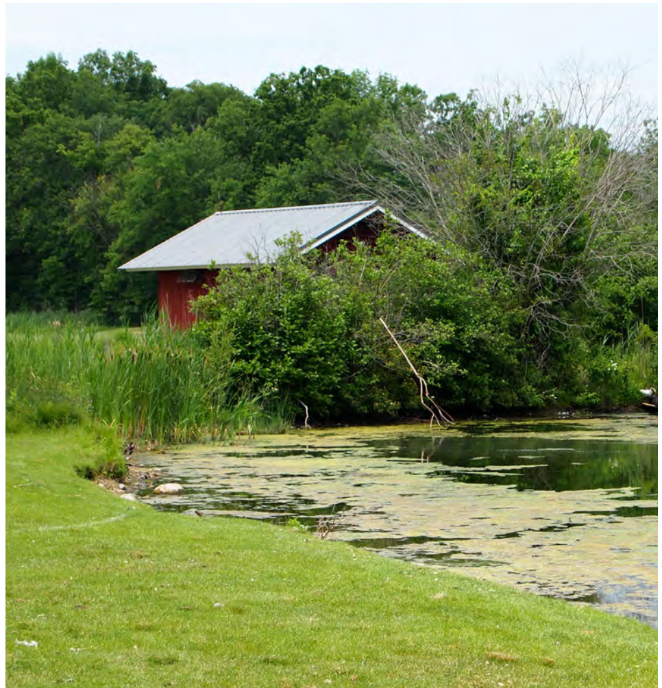
Maintenance shed overlooking artificial lake (Image 3.5.4.3)
