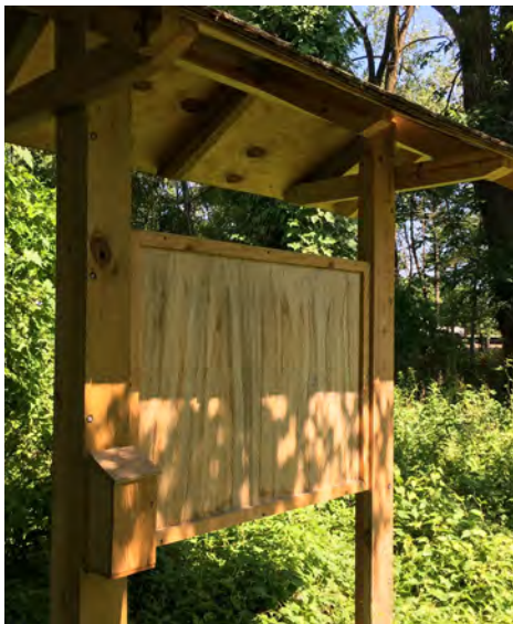
Empty signage noted as point #2 in the map (Image 3.4.1.2)
