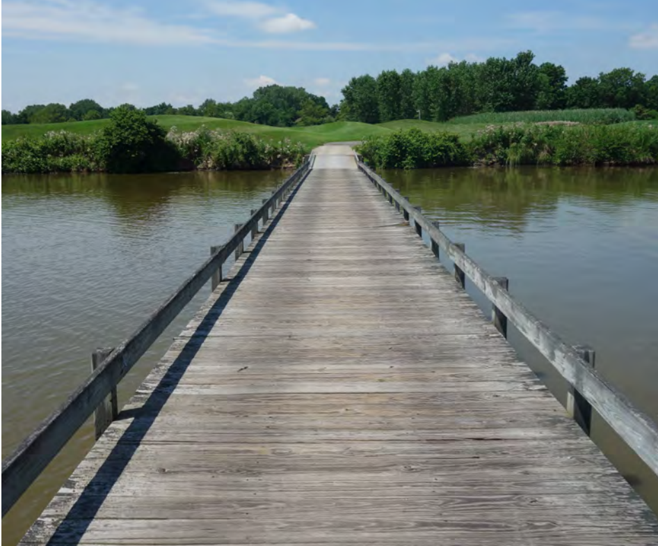
View across one of the wooden bridges (Image 3.5.5.2)
