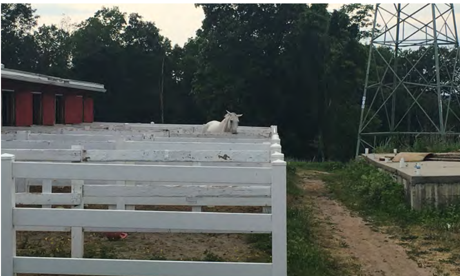
Horse pens next to electric tower in right-of-way (Image 3.2.7.3)
