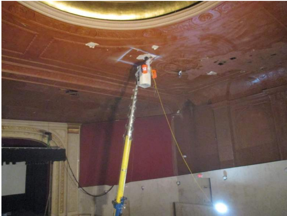
Photo 1 Plaster ceiling being cut to permit evaluation
