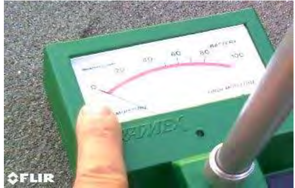
PHOTO 2 Lower Roof Section: Zero moisture detected throughout roof area.
