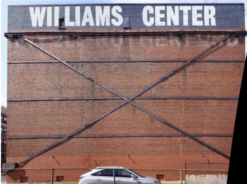
Photo 11 Steel Lateral Bracing System
