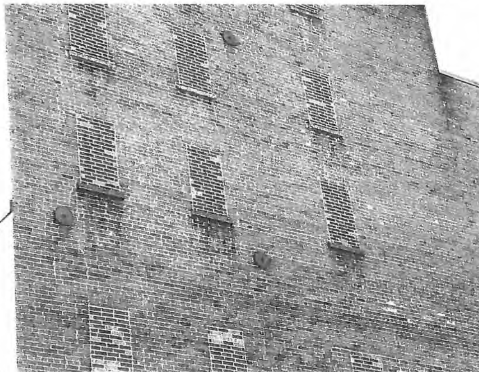
Photo 2 North Elevation at Stage (viewed from Glenn Road).
