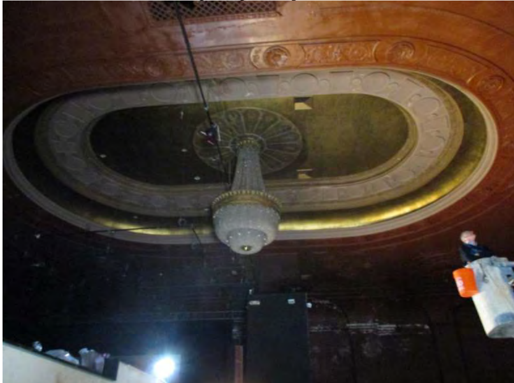
Photo 2 Chandelier within the plaster ceiling
