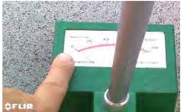
PHOTO 4 Lower Roof Section: Zero moisture detected throughout roof area.
