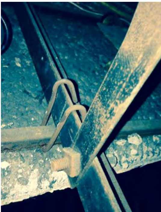
Fig. 2 Typical framing connections in the plenum of the auditorium are adequate.
