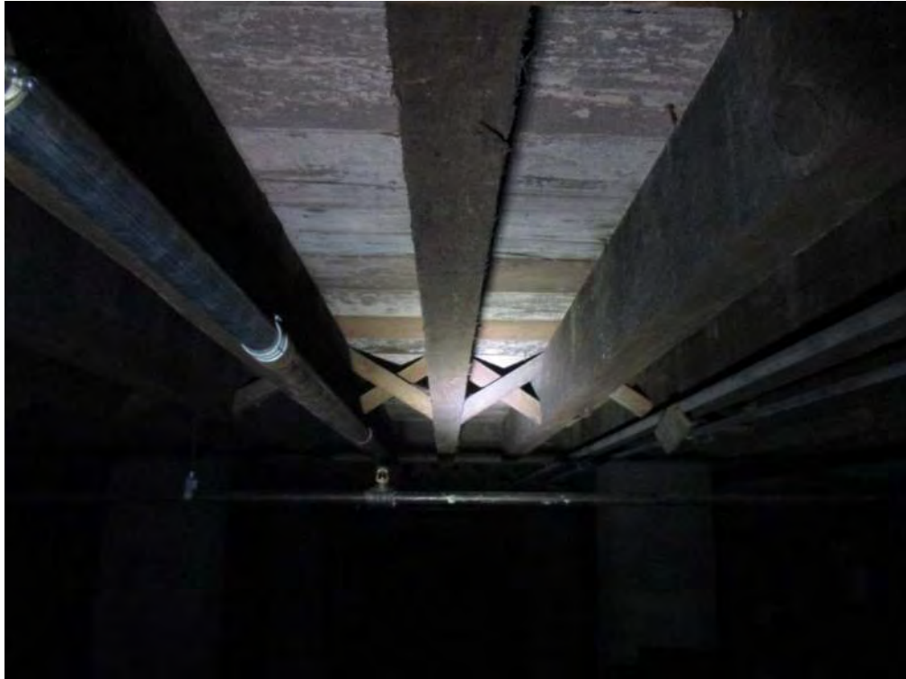
Photo 17 Floor joists under proscenium stage
