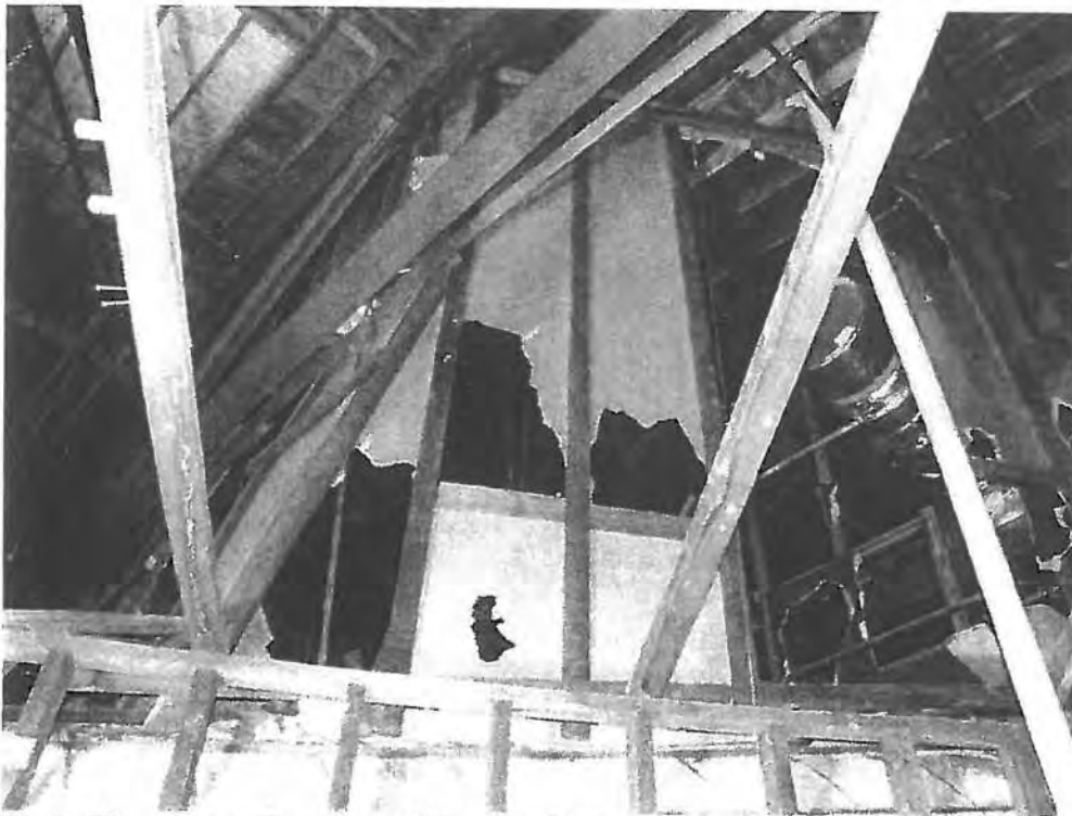
Photo 38 Another view of the metal lath and plaster ceiling from plenum along north wall. A wood stud wall has been constructed to brace the ceiling construction.
