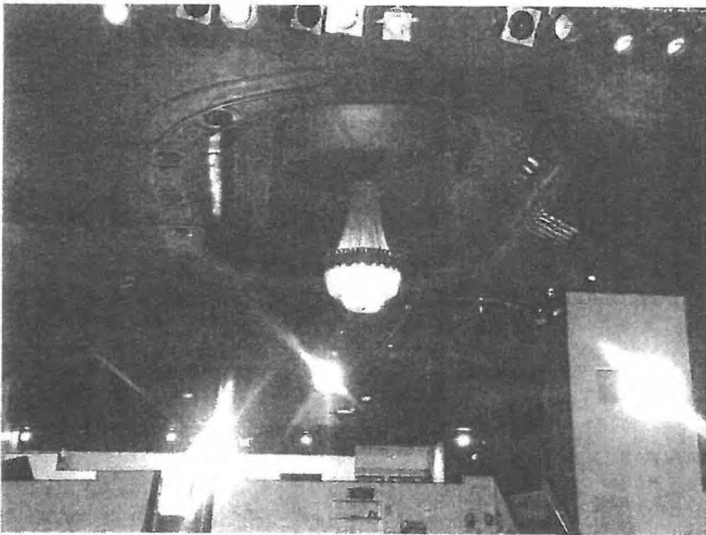
Photo 12 View of the plaster ceiling. (Viewed from downstage) Black Box theater is towards the rear.
