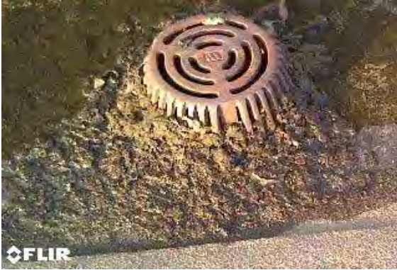
PHOTO 7 Lower Roof Section: Debris should be cleaned away at drains.
