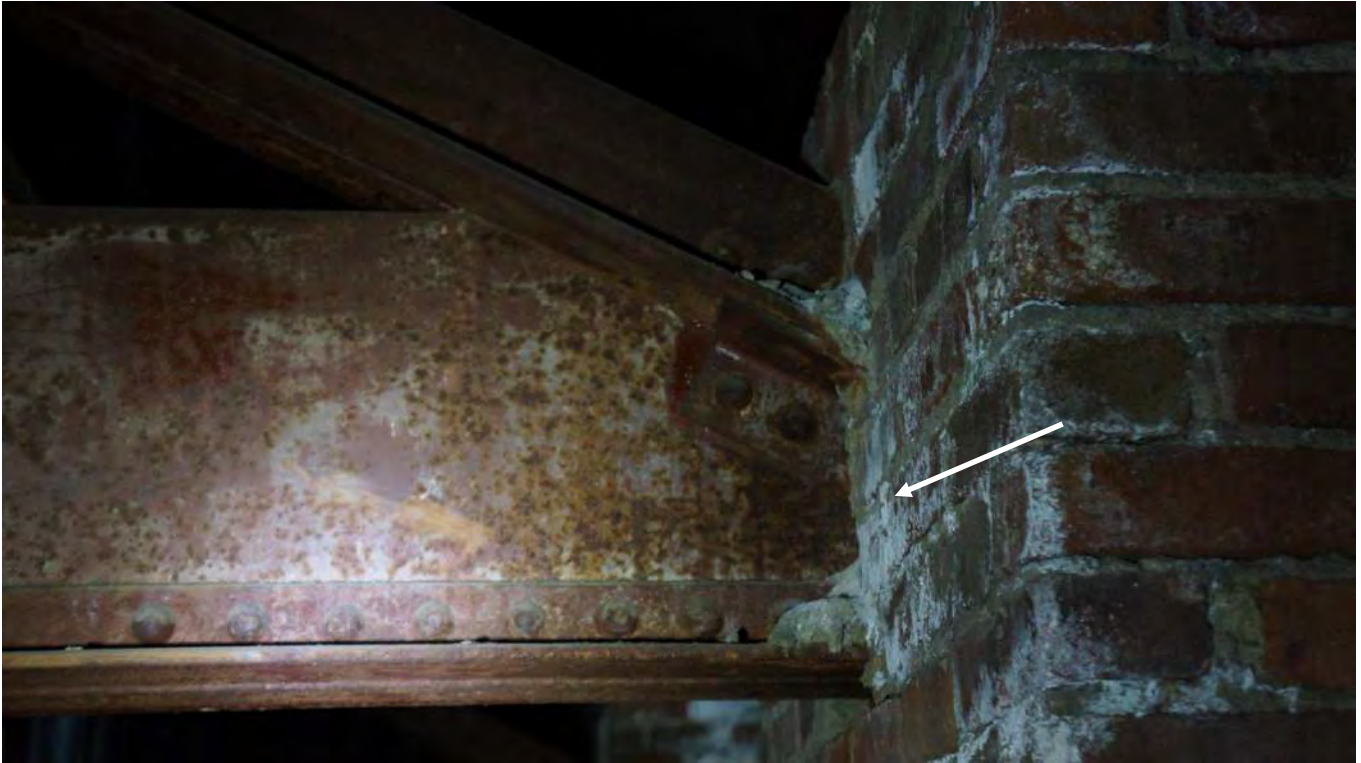
Photo 9 Masonry bearing of the roof truss
