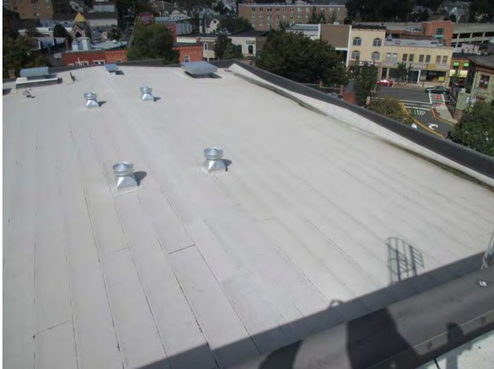
Photo 5 General view of theatre roof
